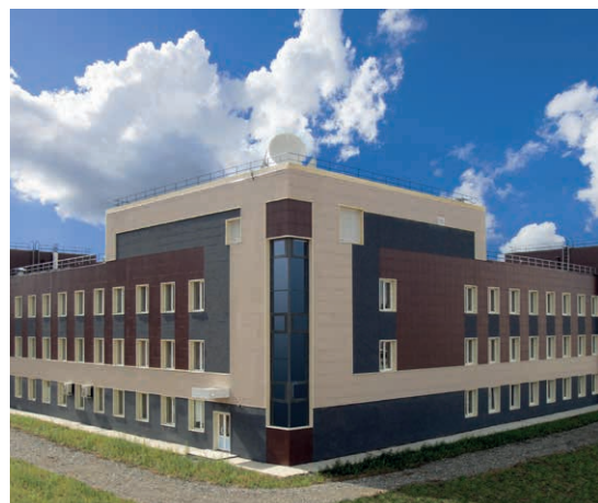
Administrative Building, Tsiolkovsky
